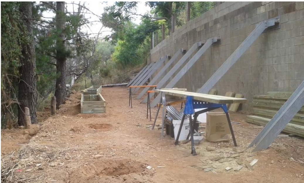
3 garden beds completed on the lower level, 27 more to go...
