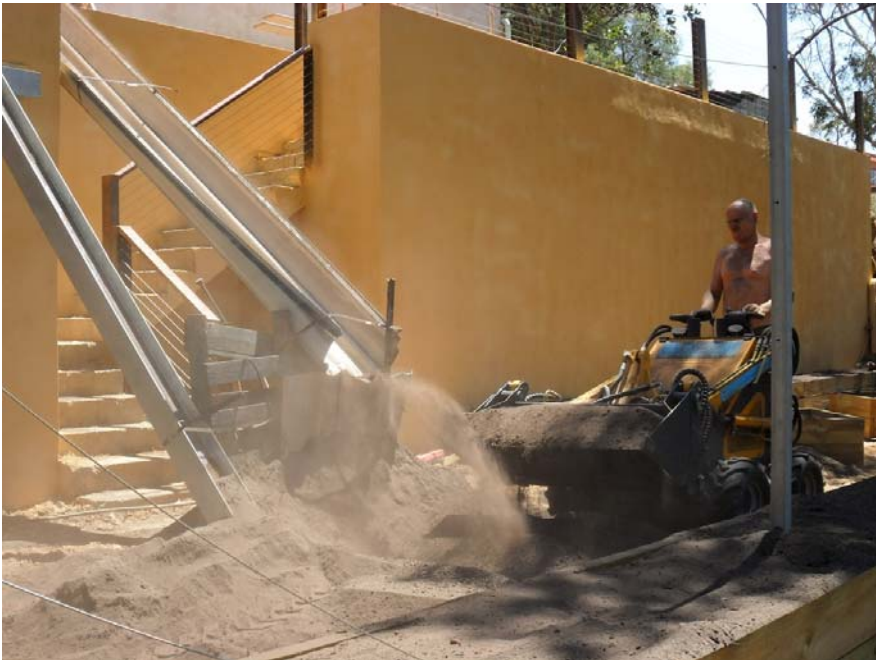
Roger moving soil at the bottom of the chute
